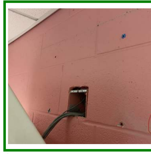
⑤ DRYWALL PATCH - Clock/Speaker Combo (EXPECT SIMILAR TO ⑥, BUT IN DRYWALL)
