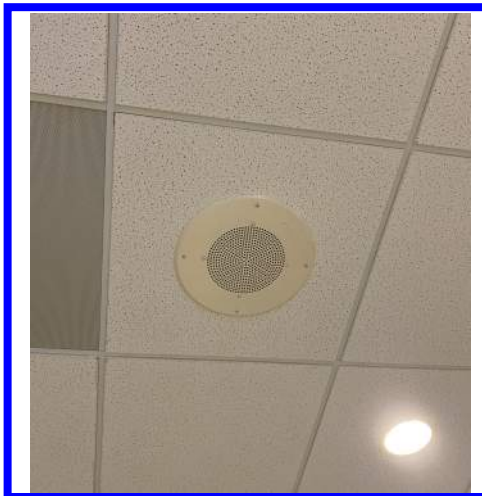
⑦ NEW ACOUSTIC CEILING TILE - 2' X 2' (TURN SPEAKER OVER TO DISTRICT)
