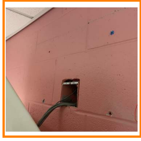
⑥ CMU PATCH - Clock/Speaker Combo
