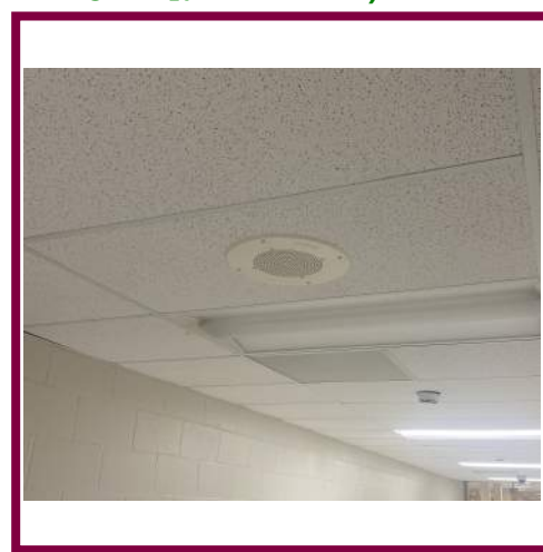
⑧ NEW ACOUSTIC CEILING TILE - 2' X 4' (TURN SPEAKER OVER TO DISTRICT)
